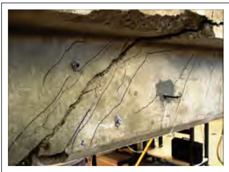
Figure 7.9 Failure mode of specimen S3-12d130s.
