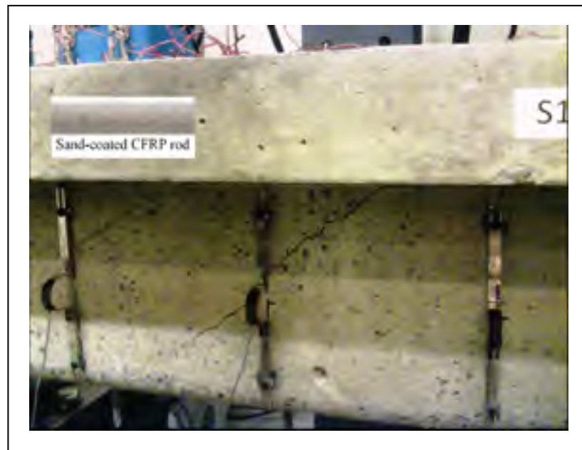
Figure 7.4 Parallel diagonal shear cracks, specimen S1-9d-260s.
