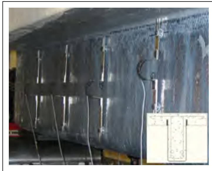
Figure 6.5 Specimen S3-EB-EFLA after the embedded FRP laminate is installed.
