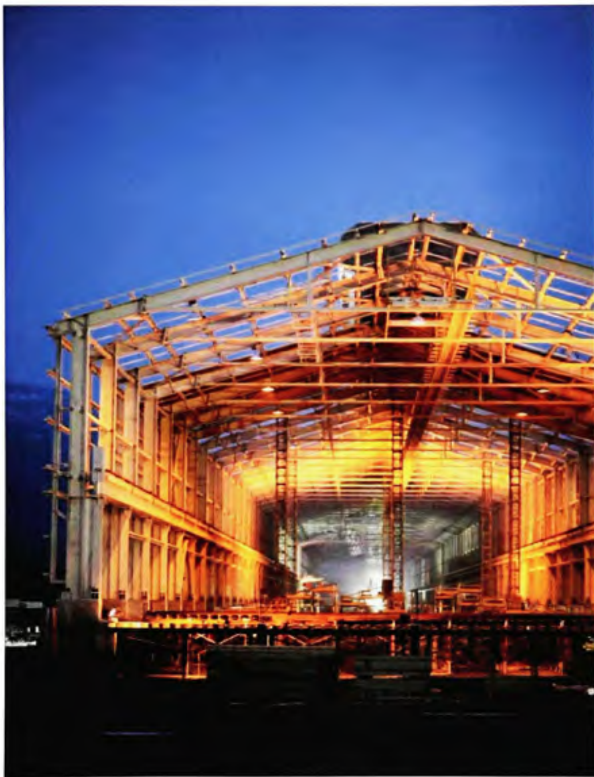
Air-Therm ventilator installed on potline building
