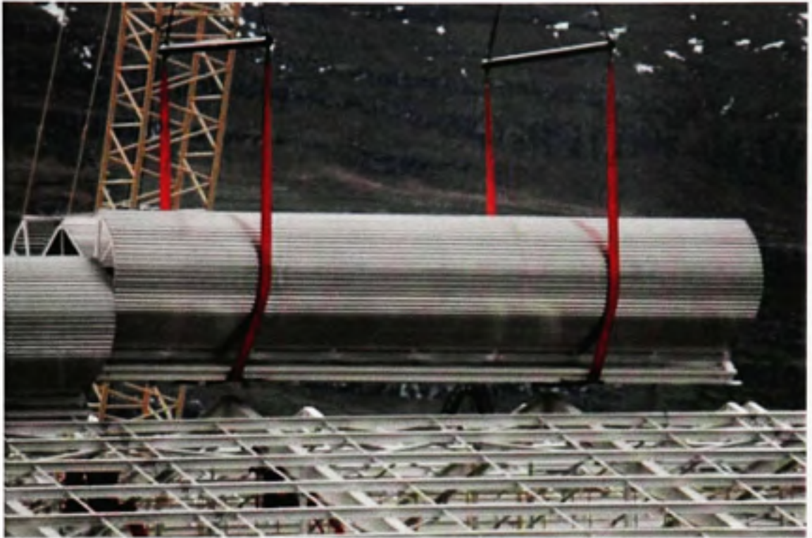
Air-Therm ventilator module being installed on potline building
