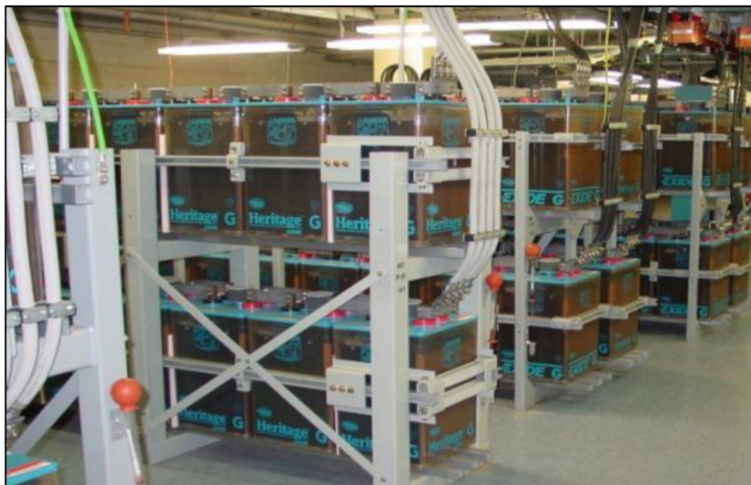
Figure 6-13 Layout of Battery Cells Room Taken from IEEE – Lead Acid Battery Fundamentals Presentation
