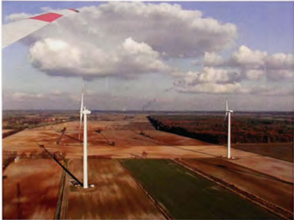
Figure 3.3 Wietmarschen site located in Germany.
