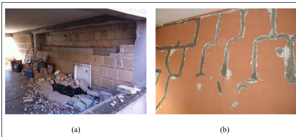
Figure 1.2 Damage to (a) infill walls and (b) internal partition after M_w 4.9 earthquake in Italy, 2013
