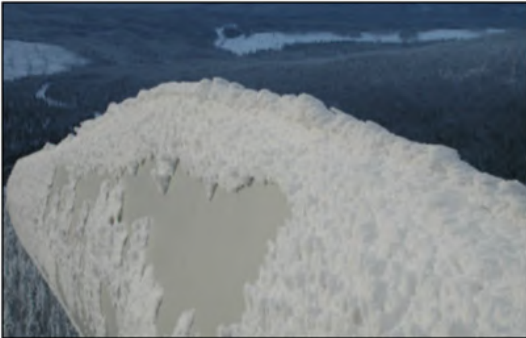
Figure 1.4: Frosted ice accumulated on the WT Blade's shoulder (photo by LM Wind Power Group) (kaupunki, 2011)
