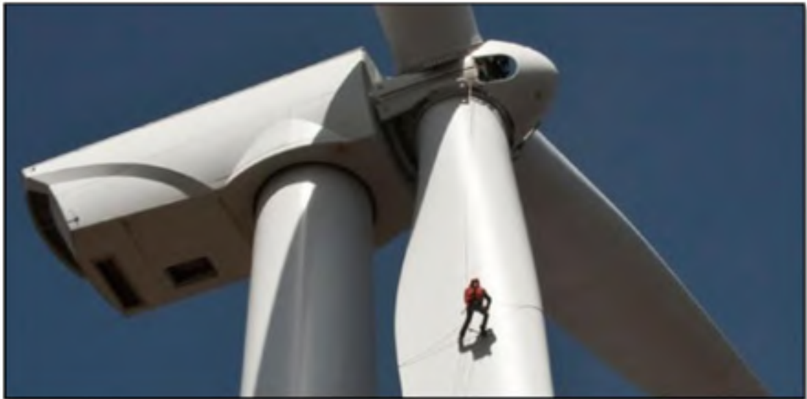
Figure 3.26: Access to the blades' surfaces by access man hole in the wind turbine hub (source : http://www.frontierpro.com )
