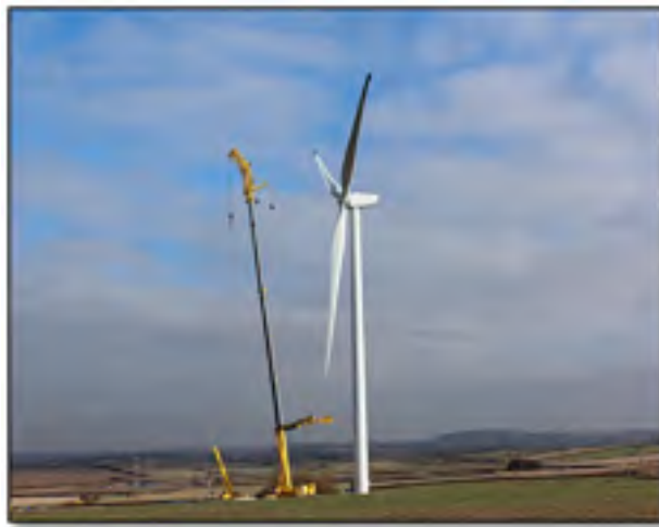
Figure 3.24: RE POWER MM 92 & Crane Withdraws (source: http://myrenaultzoe.com/index.php/2013/02/17/ : image: T. Larkum)
