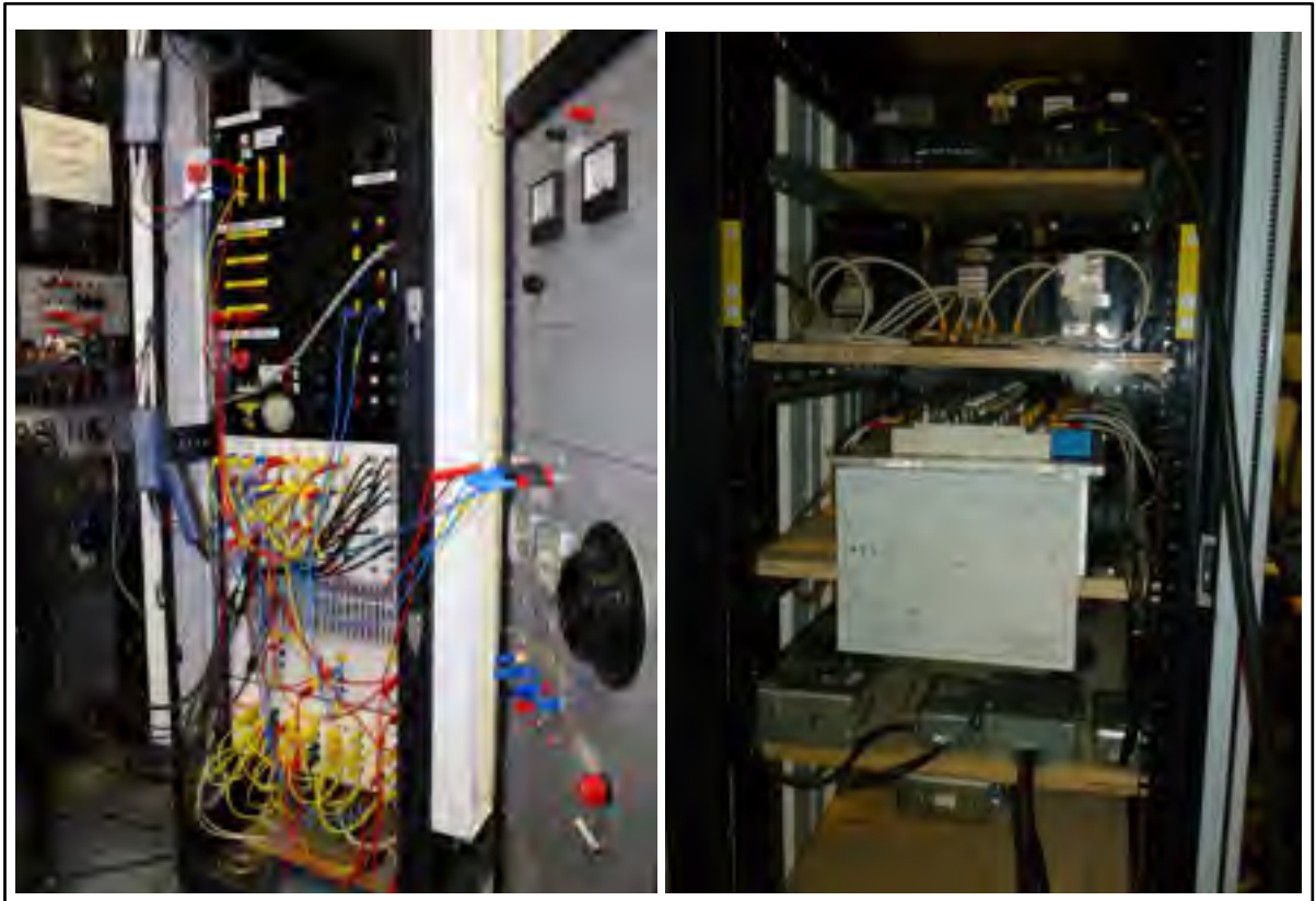
Figure-A III-1 The Transformerless Hybrid Series Power Active filter setup
