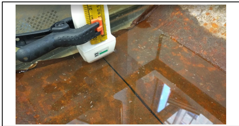
Figure 3.10 Array setup above the groove under inspection
