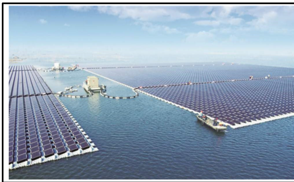
Figure 1.2 Centrale photovoltaïque offshore Tirée de Sungrowpwer (2018)
