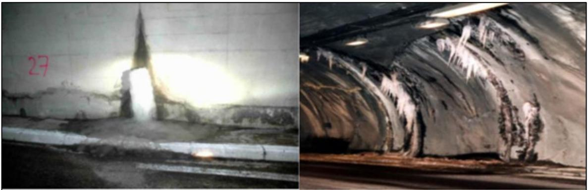
Figure 1.1 Expansion joint and ice in the tunnel
