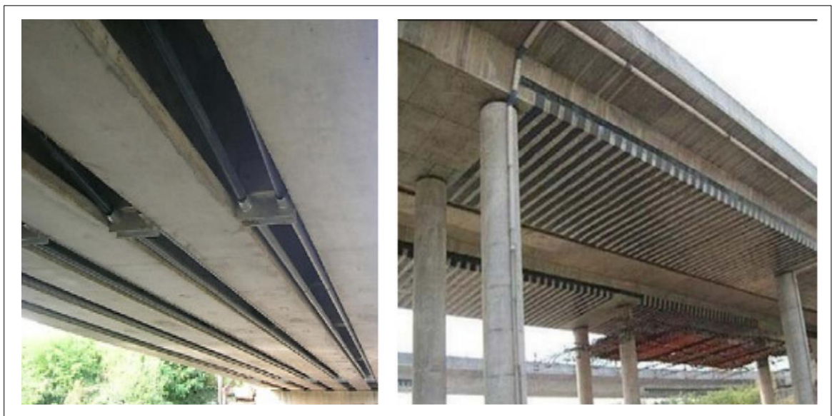
Figure 1.3 Bridge strengthening with EB-FRP systems Taken from Siddika et al. (2020)
