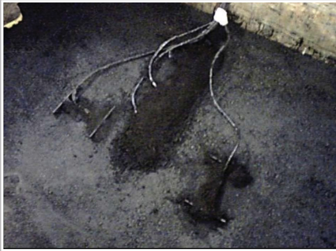
Figure 1.14 H-type asphalt strain gauges installed within the asphalt layers Taken from Correia et al. (2018)
