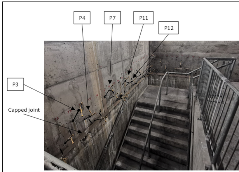
Figure 3.1 Capped construction joint used for the in-situ test
