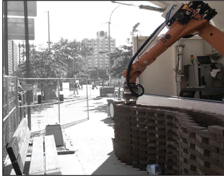
Figure 1.20 Case Study for the Design and Production of Concrete ‘Pop-up’ Structures Taken from Vazquez & Jabi (2015, p.9)
