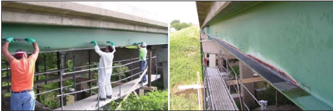
Figure 1.10 Retrofitting steel bridge elements - Pottawattamie County, Iowa Taken from Phares, Wipf et al. (2003, p. 10)
