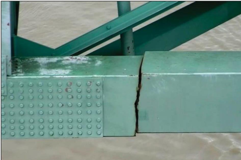
Figure 1.2 Cracked element of I-40 bridge Taken from CBC News Staff (2021)
