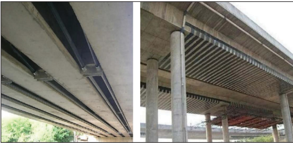
Figure 1.6 Retrofitting of a concrete bridge using the EB FRP technique Taken from Siddika, Mamun et al. (2020, p. 2)
