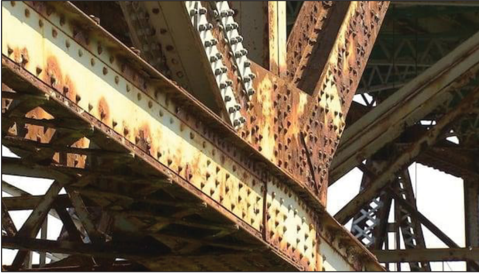
Figure 1.1 Corroded elements of Mercier Bridge Taken from CBC News Staff (2011)
