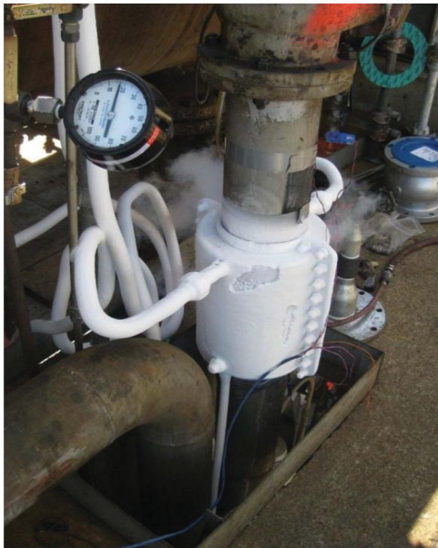
Figure 1.10 Frost developing on jacket during freezing operation
