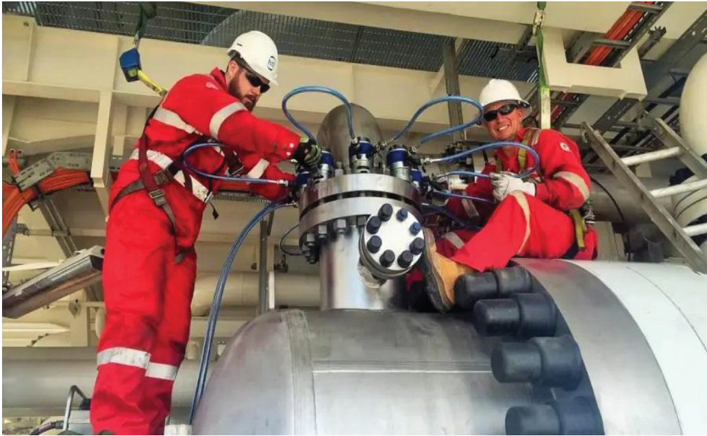
Figure 1.9 Heat exchanger bolt stress measurements
