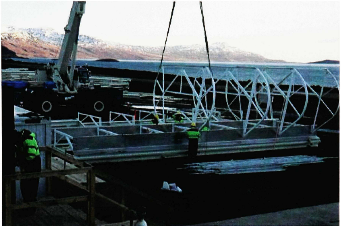
Air-Therm ventilator module being assembled on the ground: due to barcode system module utilizing this system were assembled faster and utilizing less labour
