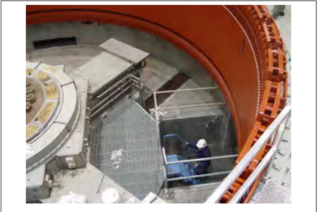
Figure 2.3 Stator of a large synchronous machine
