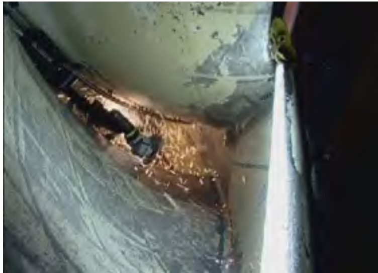
Figure 1-2 SCOMPI during on-site maintenance (Charles Gagnon, 2010)
