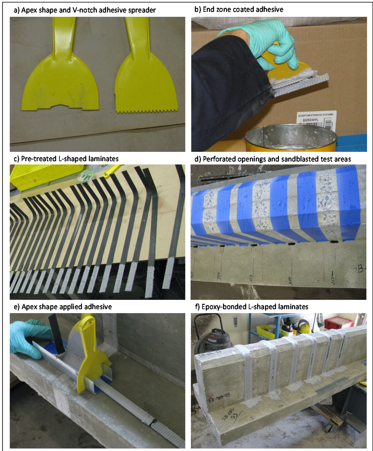
Figure 5.2 Step-by-step procedure for CFRP L-shaped laminates application
