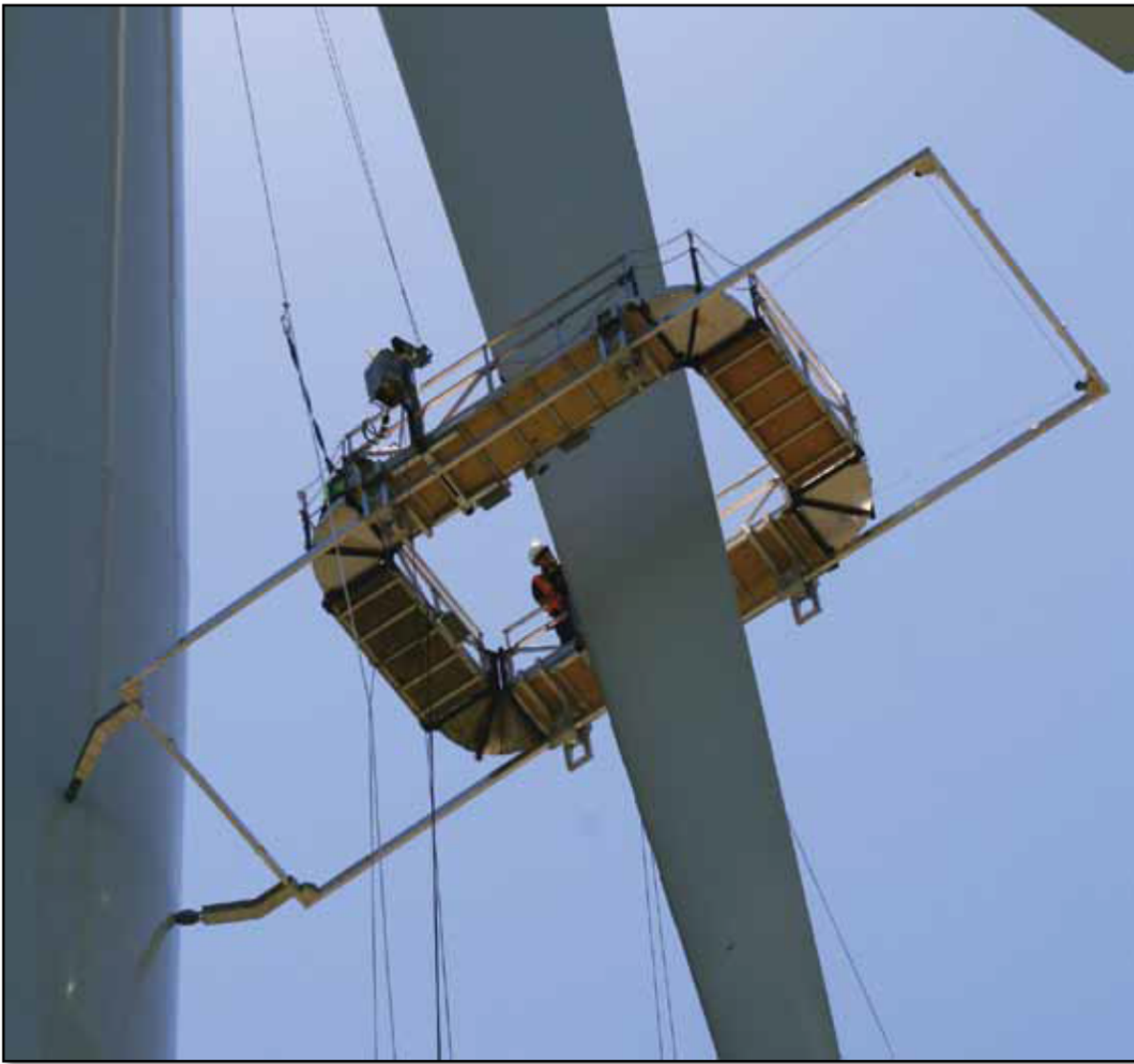
Figure 3.25 : Suspended access equipment for Wind Turbine ( www.spiderstaging.com )
