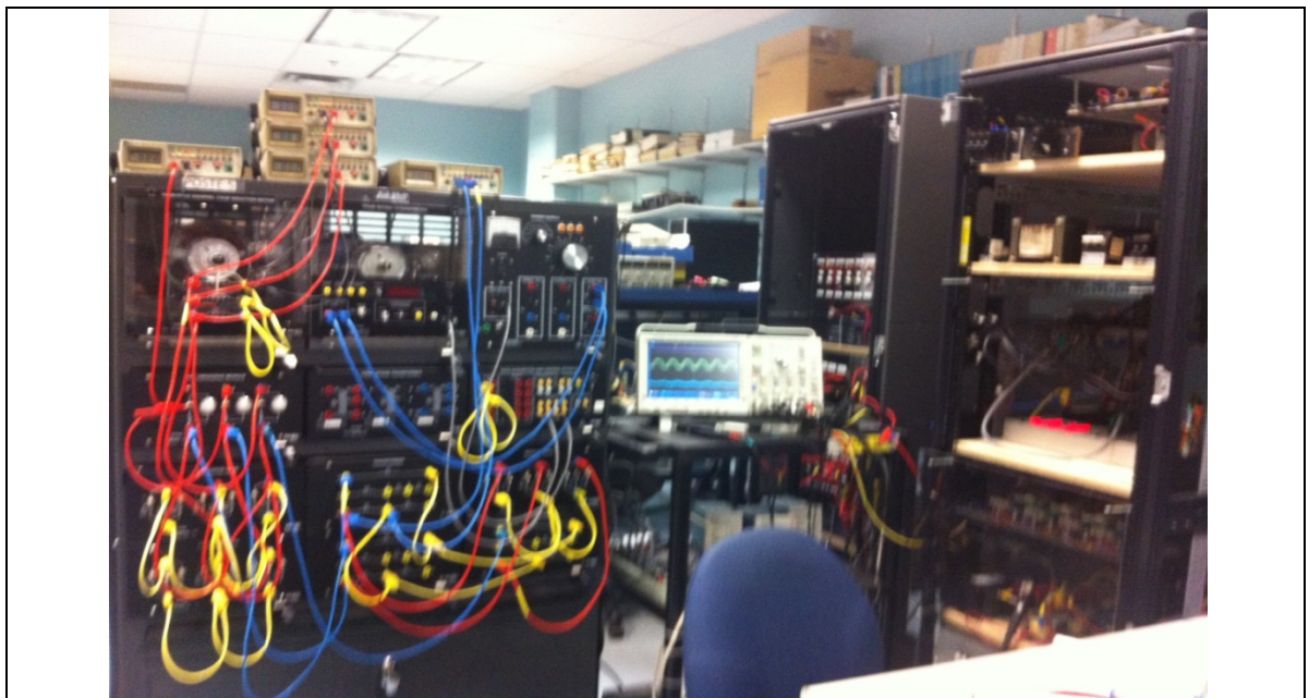
Figure A.1.3 Experimental Setup for hybrid standalone system based on PV array and MHP driven fixed speed SCIG
