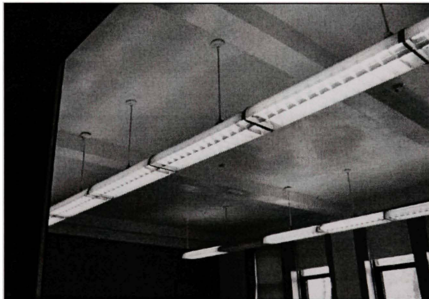
Figure 3.27 Luminaires suspendus.
