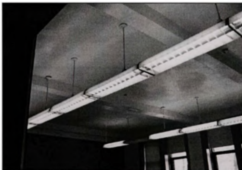
Figure 3.27 Luminaires suspendus.
