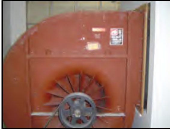
Figure 3.3 Double impeller centrifugal fan
