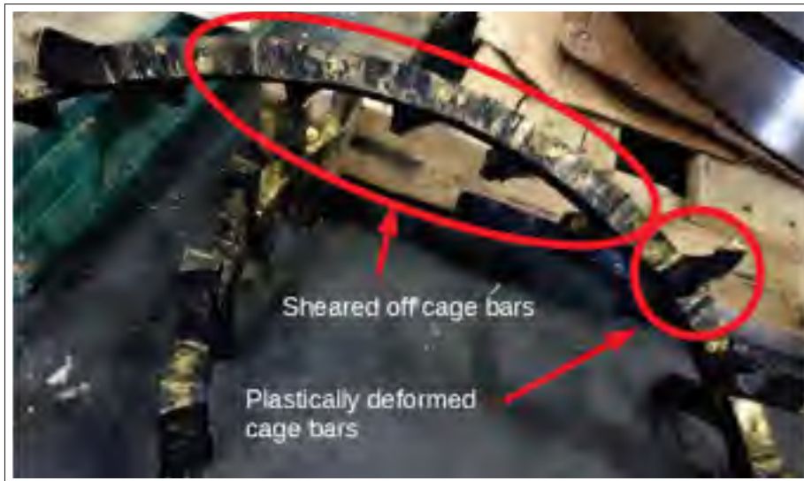
Figure 4.5 Pictures of main bearing cage parts showing the damage for case study A.
