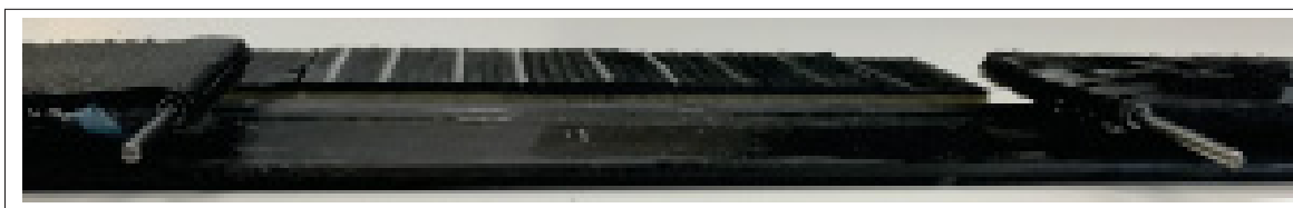
Figure 3.25 Pin Loaded Strap installed on CFRP beam
