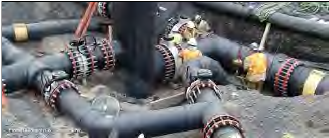
Figure 0. 3 On-field HDPE flange installation
