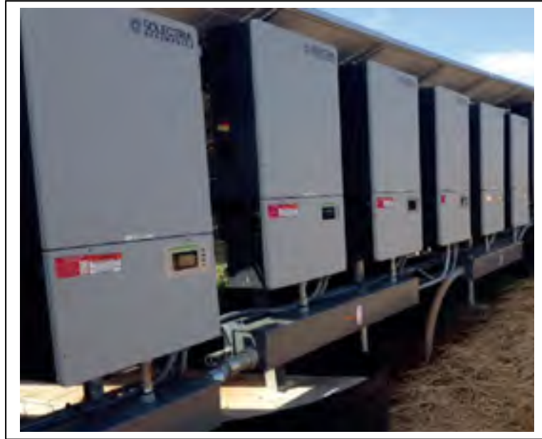
Figure 6-11 36 kW DC - AC Power Inverter - PV Arrays Taken from Yaskawa Solectria Solar PVI 36TL Technical Datasheet (2017)
