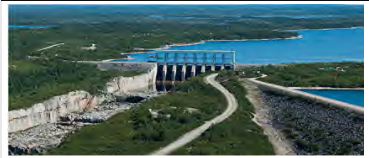
Figure 4-3 Robert-Bourassa (formerly La Grande-2) Hydropower Generation station Taken from Hydro Québec – Robert Bourassa Generating Facility (2018)
