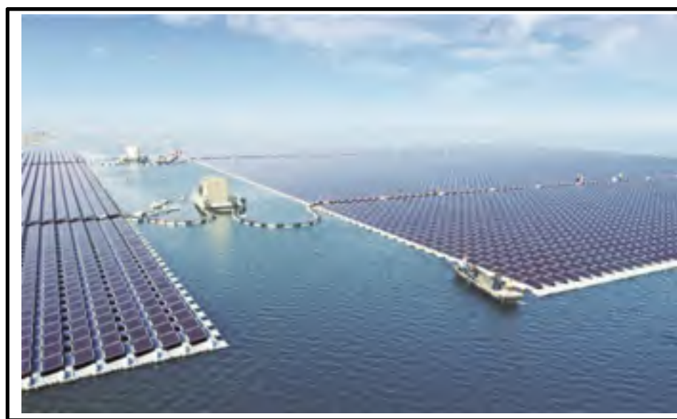
Figure 1.2 Centrale photovoltaïque offshore Tirée de Sungrowpwer (2018)
