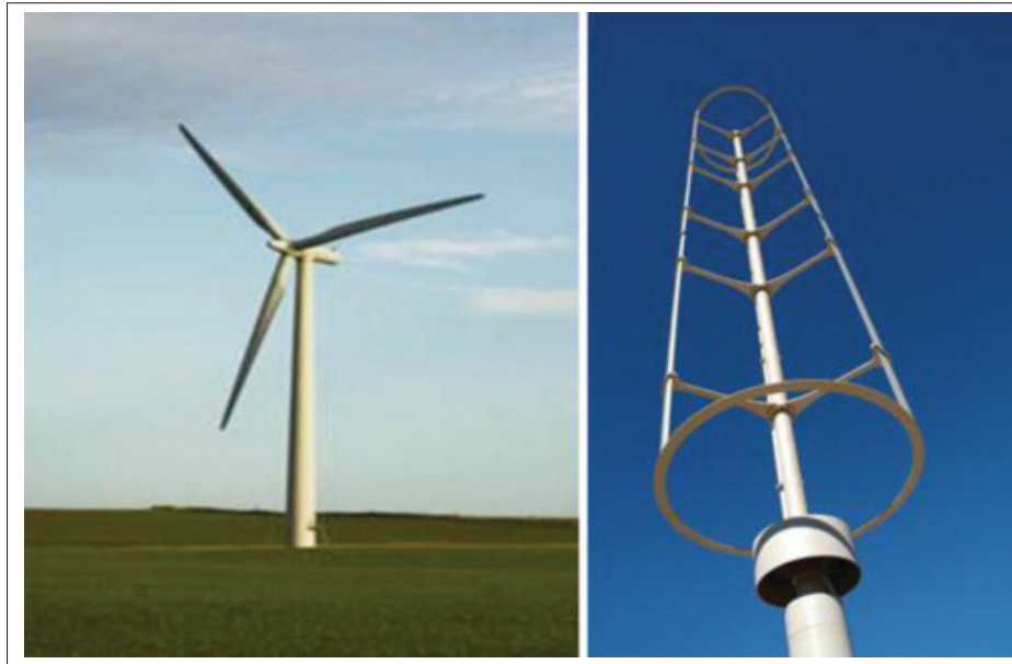
Figure 0.6 HAWT (left) and VAWT (right)
