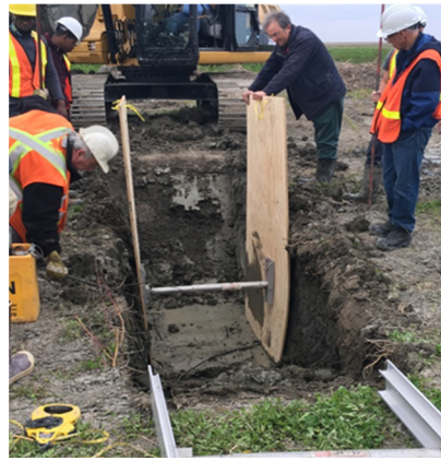
(b) It takes time and manpower to arrange the shoring in this type of soil
