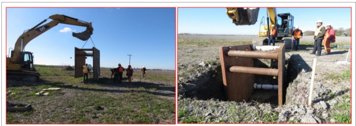
Figure 3.10 Installation of the first (lower) trench box into the trench
