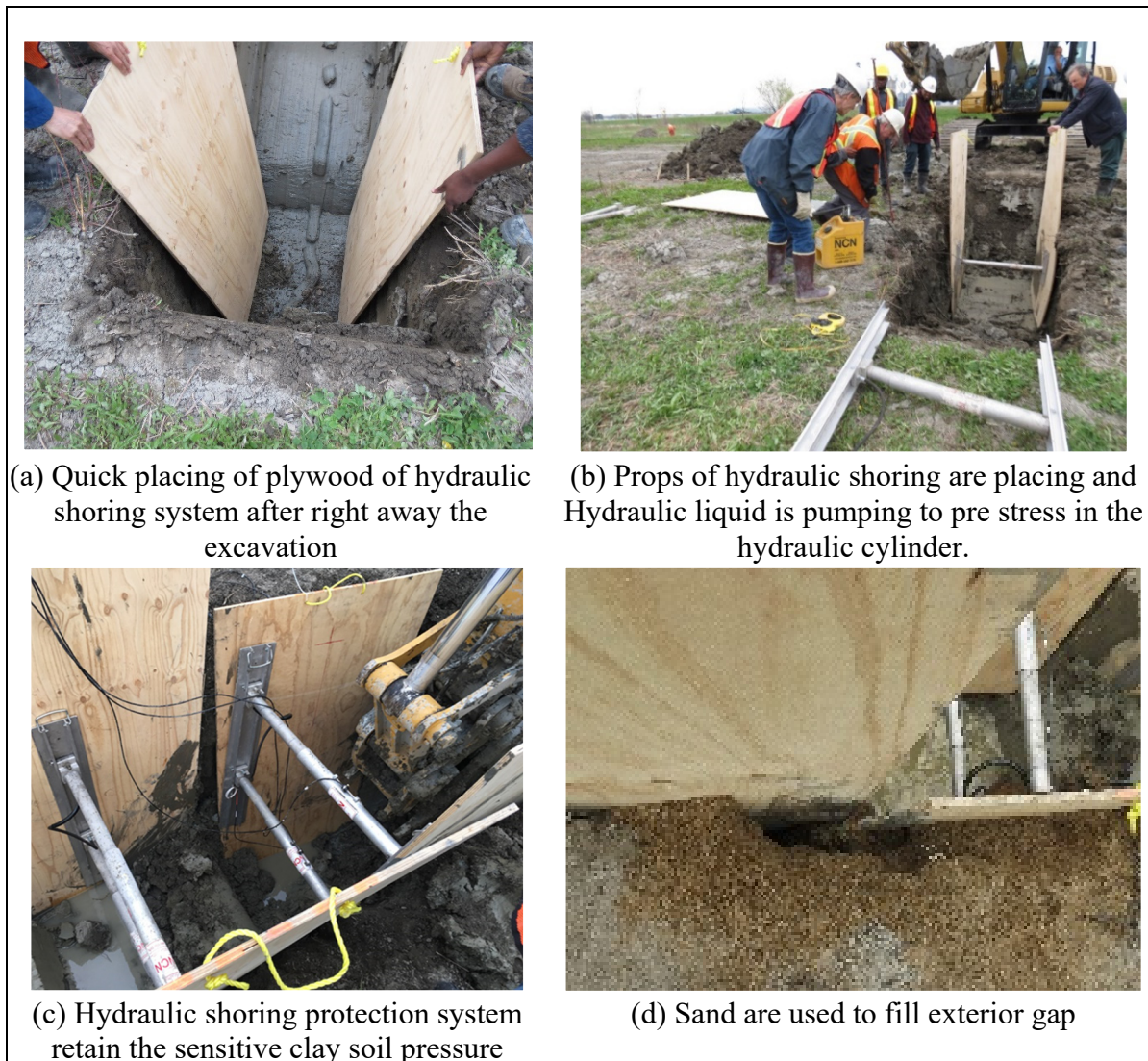
Figure 6.6 Detail installation process of Hydraulic shoring with Plywood in a shallow trench of soft and sensitive clay
