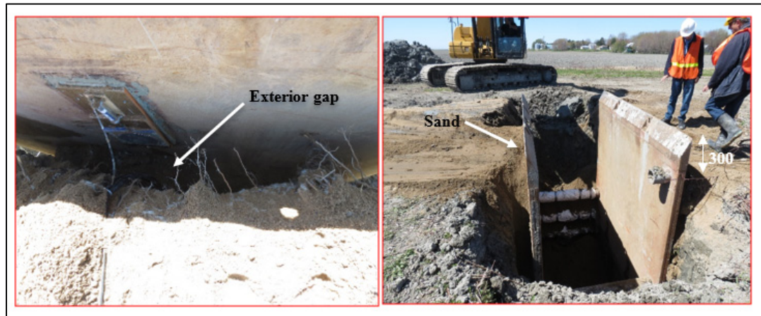
Figure 3.13 Sand was used to fill the space between the shoring exterior wall and the surrounding soil
