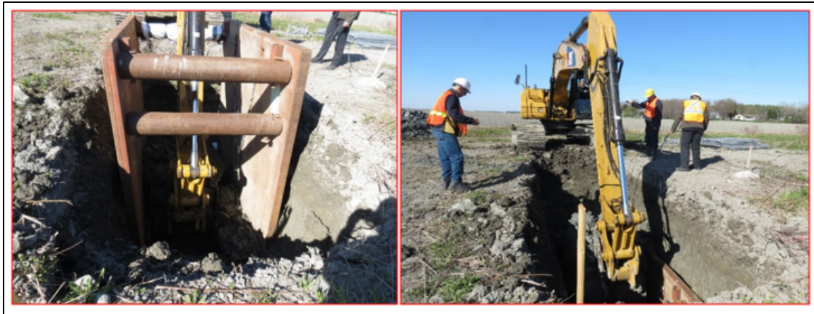
Figure 3.11 Excavation continued to make room to accommodate the second (upper) trench box in the trench
