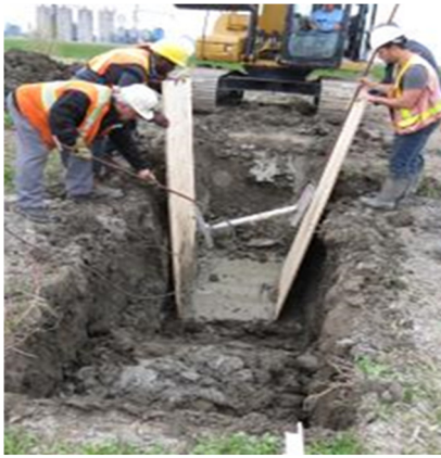
(a) Many people are required to installed this shoring system in this soft and sensitive clay
