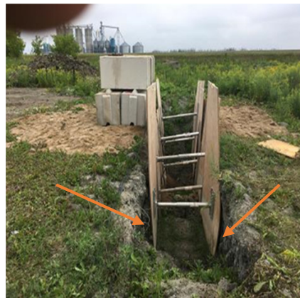
(d) Rain water washed away the soil between the plywood and shoring soil
