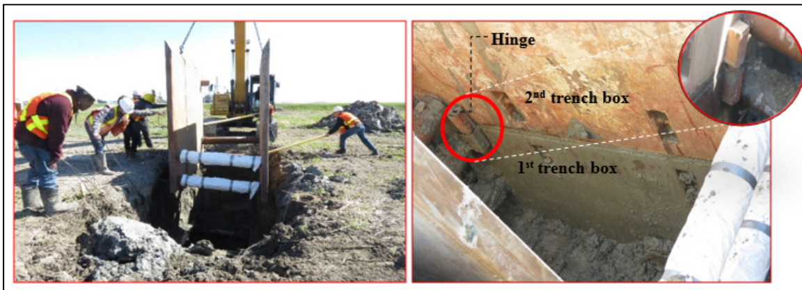
Figure 3.12 Second (upper) trench box is being placed on top of the first (lower) box in the trench
