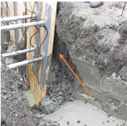
(c) Spotted soil cave-in to the trench after the installation of shoring system
