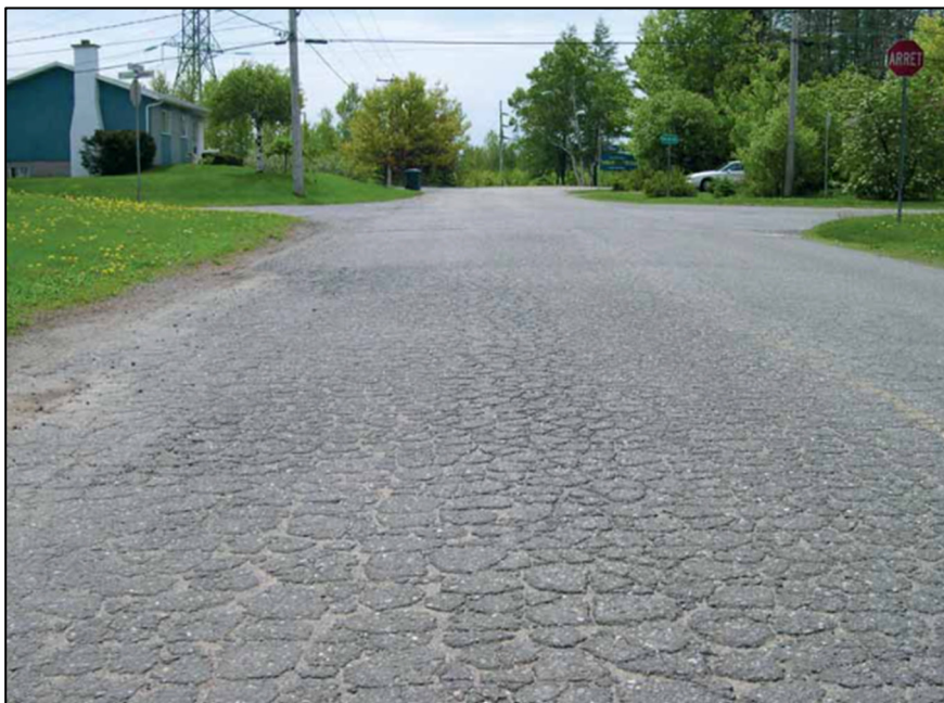
Figure 1.10 Alligator cracks
