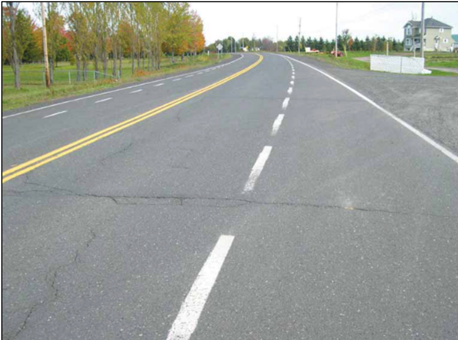
Figure 1.8 Transverse cracks
