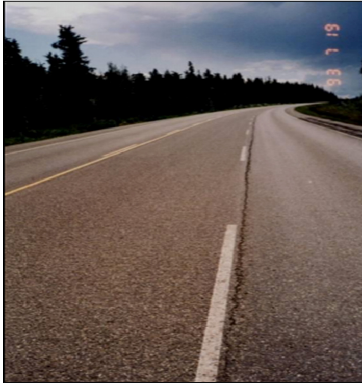
Figure 1.13 Longitudinal joint cracking Taken from Pavement Surface Condition Rating Manual BCMoT (2020)
