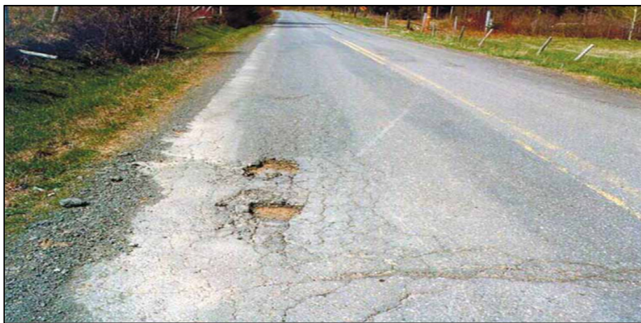
Figure 1.18 Disintegration/Potholes
