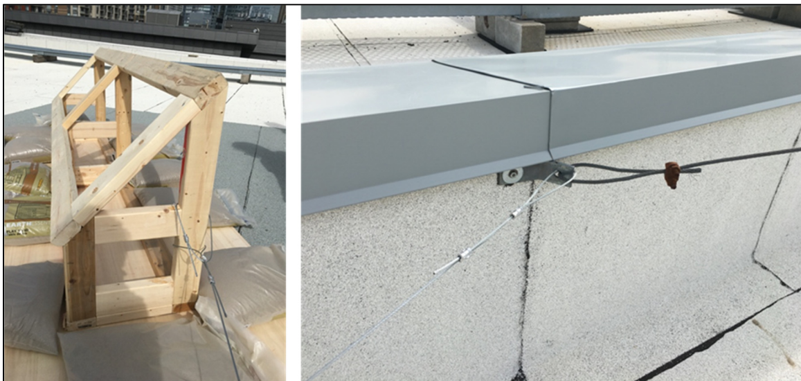
Figure 2.12 Structure fixation
