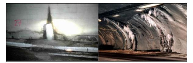
Figure 1.1 Expansion joint and ice in the tunnel Taken from CETU (2015)
