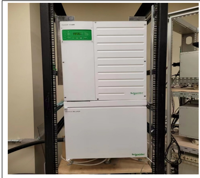
Figure 2.8 Schneider XW Pro 6848 hybrid Inverter
