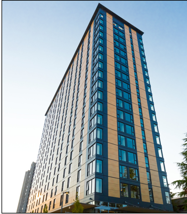
Figure 1.20 Brock Commons Tallwood House Tirée de NaturallyWood.com
