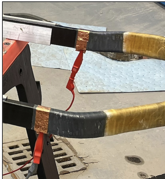
Figure 6.6 Picture of one of the guard electrodes installed on coil 07
