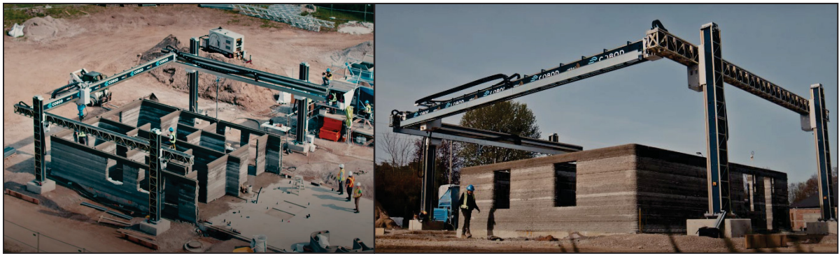
Figure 2.16 Progressive stages of 3D printing construction Taken from Nidus3D (2024)
