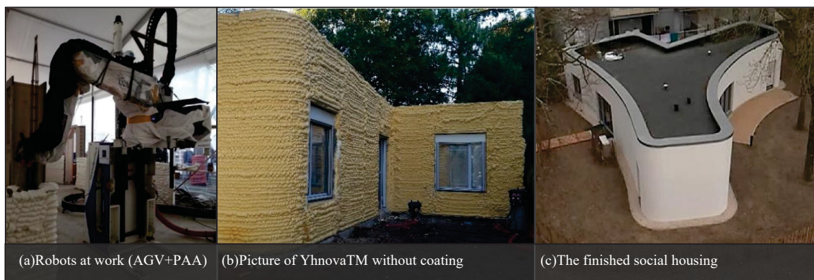
Figure 2.7 The Batiprint3D™ process from Start to finish Taken from Furet et al. (2019, p. 63)
