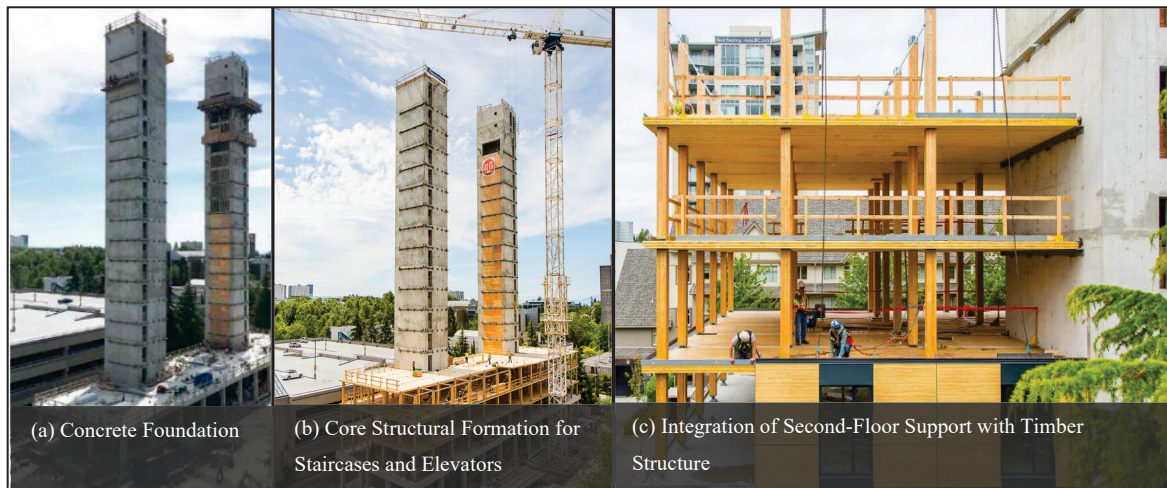
Figure 2.18 Structural foundation and core construction of Brock Commons Taken from Acton Ostry Architects Inc. & Forestry Innovation Investment (2017)
