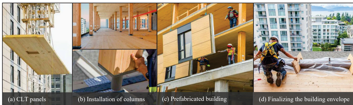
Figure 2.19 Stages in the construction of the Brock Commons building envelope Taken from Acton Ostry Architects Inc. & Forestry Innovation Investment (2017)
