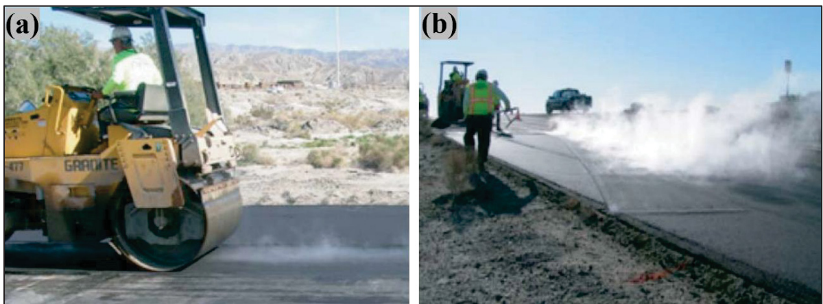
Figure 1.2 Steams emitted from WMA (a) and HMA (b) during compaction
